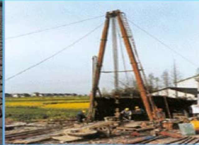
Deep groundwater pumping
